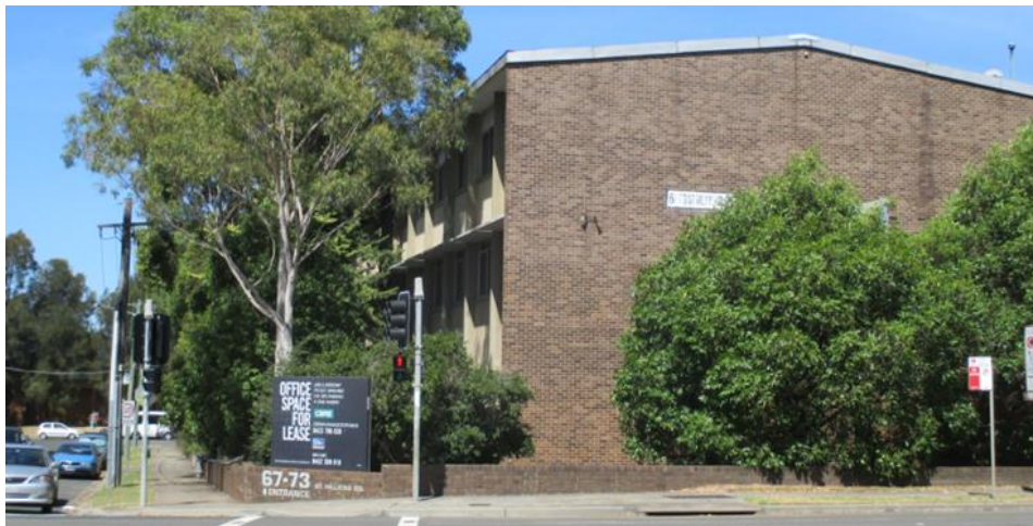
Figure 2- Western side of the office building (viewed from St Hilliers Rd).
