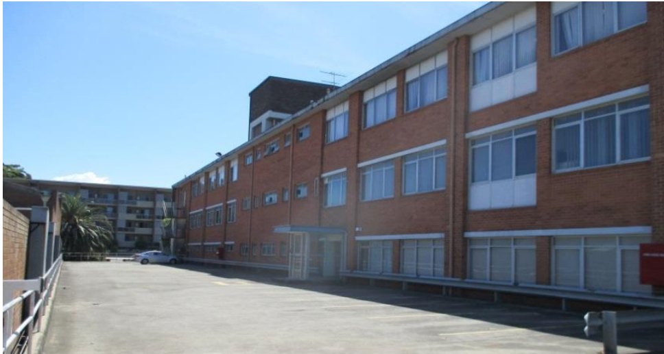
Figure 5- Upper level car park. As viewed from the eastern / Percy Street end of the car park.
