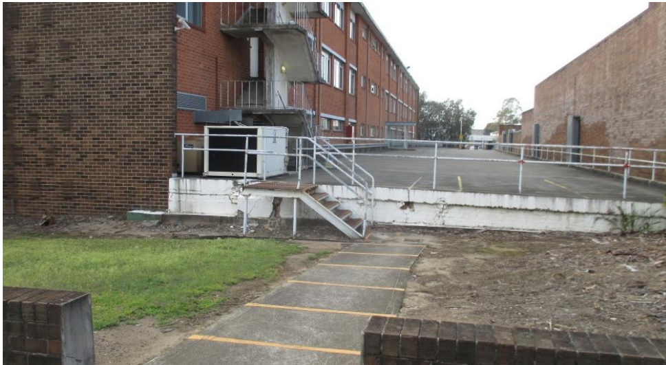
Figure 6- Upper level car park. As viewed from the pedestrian walkway along St Hilliers Road (western end of the site).
