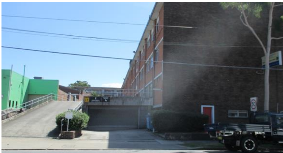
Figure 3- View of the eastern side of the office building and the lower and upper car park access driveway (viewed from Percy St).
